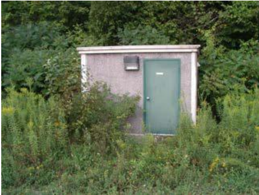
Photo 5 – View of a typical Control Valve (CV) Hut. Vegetation becomes re-established around the huts relatively quickly. GEC 2018-08-26
