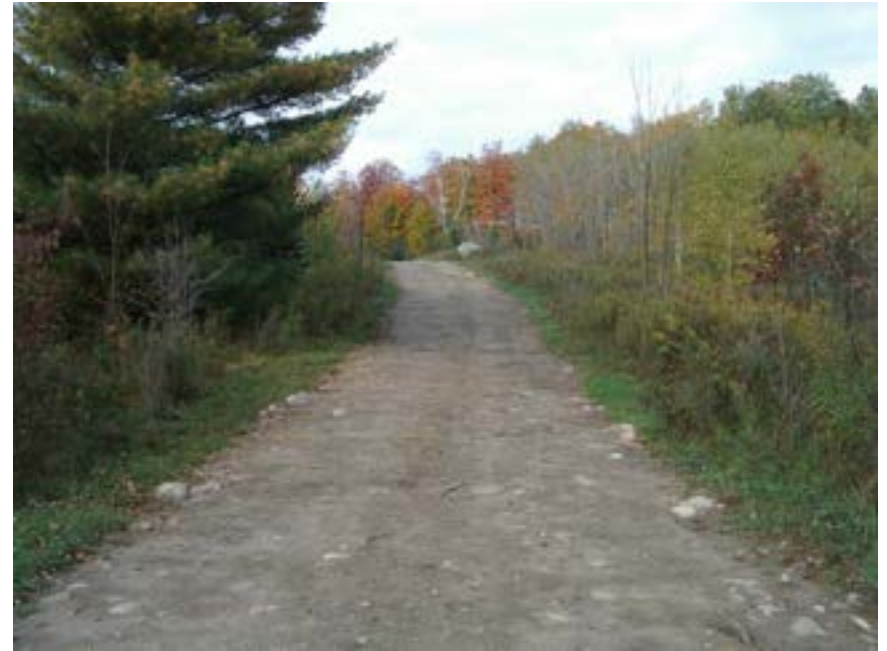
Photo 8 – Second view showing recently buried feeder lines leading to Recharge Wells RW203C, RW203D, RW204C and RW204D, closer to Sixth Line. GEC 2012-10-09
