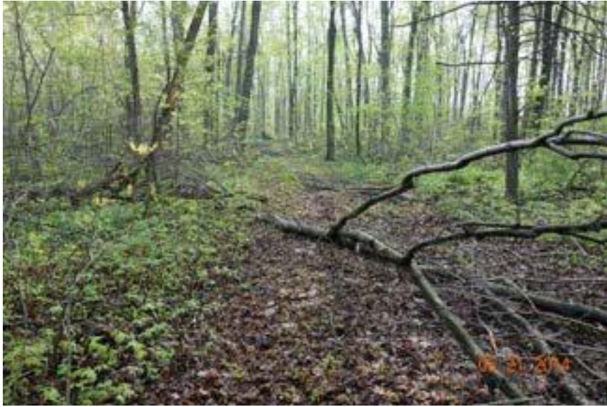
Photo 21 – View of the feeder line leading to Recharge Well RW316C, taken 3 years after the feeder line was buried in 2011. Note the woody debris. GHD 2014-05-21
