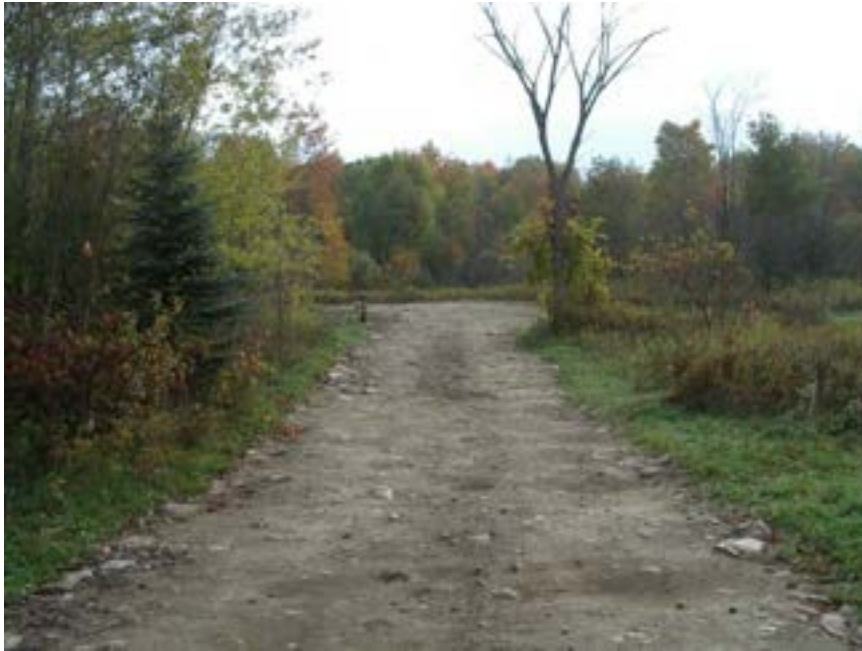
Photo 7 – View showing recently buried feeder lines leading to Recharge Wells RW203C, RW203D, RW204C and RW204D, closer to Sixth Line. GEC 2012-10-09
