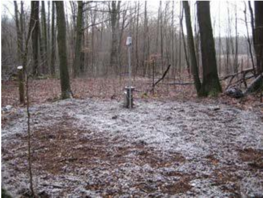
Photo 29 – View showing Recharge Well RW316C shortly after installation in late 2012. Note the 15-20 cm deep layer of fresh wood chips that were placed on the disturbed area.
