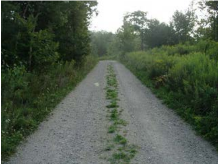
Photo 3 – A view of the East Cell watermain and driving access. In areas where the alignment crossed through old field areas, the shoulder and safety berm (on the right side of the access in this photo) were seeded with a standard MTO seed mix. The extraction area is off to the right.
