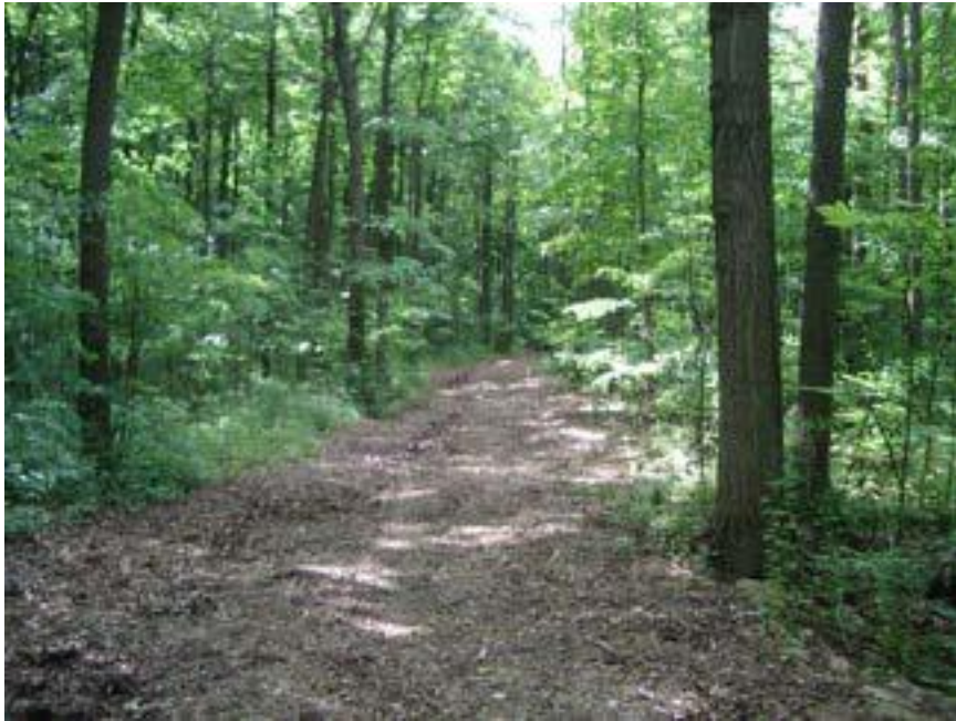
Photo 15 – View of buried feeder lines leading to the RW317 series of recharge wells. GEC 2012-05-31
