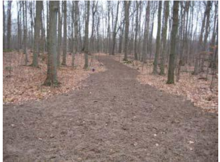
Photo 14 – This is the same view of buried feeder lines to Recharge Well RW317D, after restoration. The 15 to 20 cm deep layer of wood chips helps to prevent the establishment and spread of invasive groundcover species such as Garlic Mustard ( Alliaria petiolata ). GHD 2012-11-30
