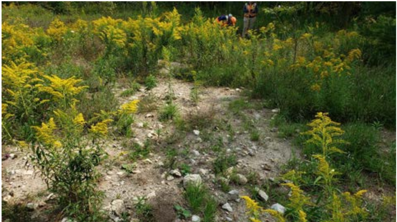
Image 25: Overview of area with fill capped test pits; facing east, September 15, 2020.
