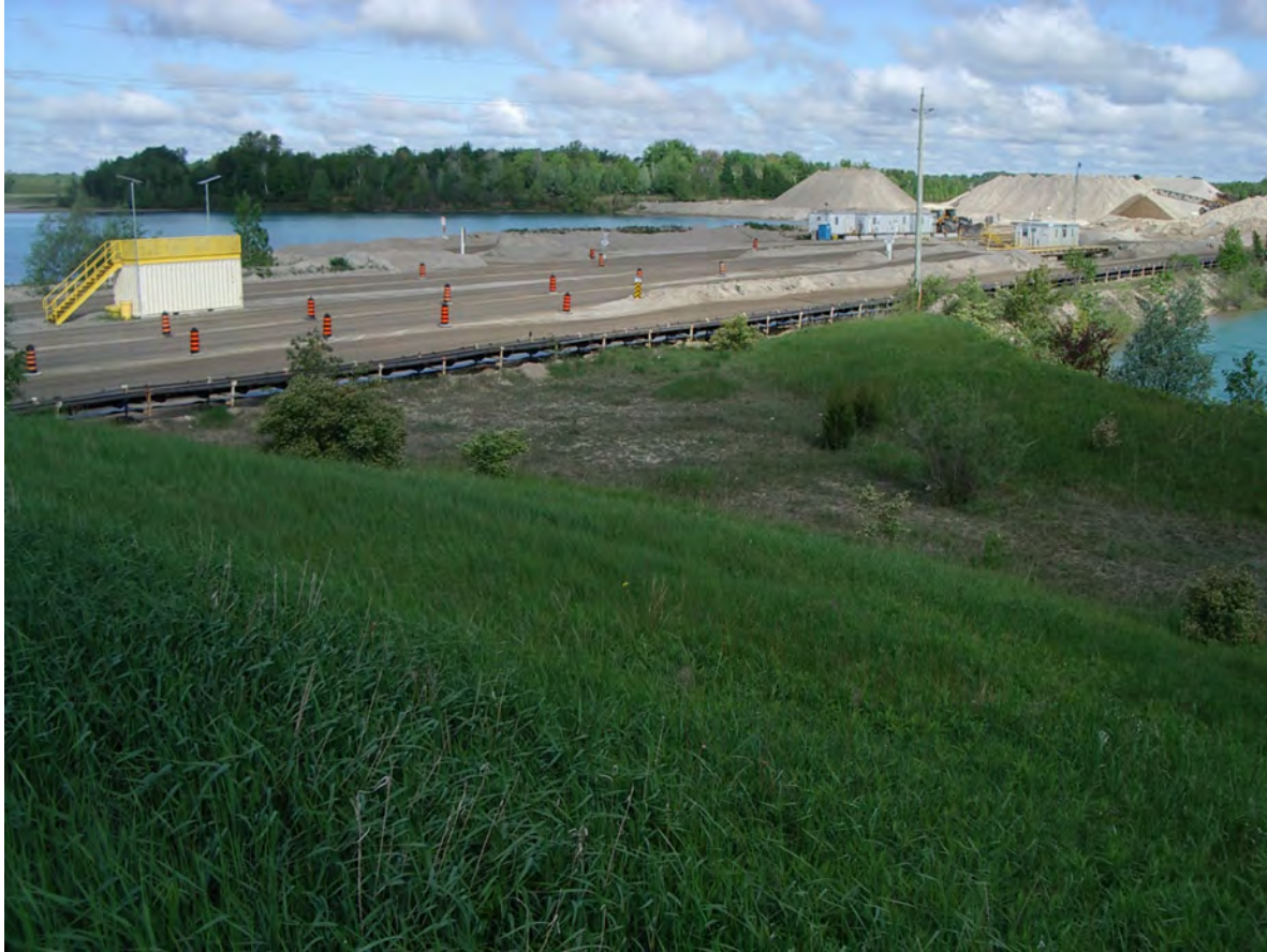
Photo 9: View looking northwest from atop the Phase 1 berm. The weigh scales to the right are in the existing approved extraction area. The land in the foreground and the tarping station (yellow/white structure) are in the proposed SPA extraction area. GEC 2022-05-28
