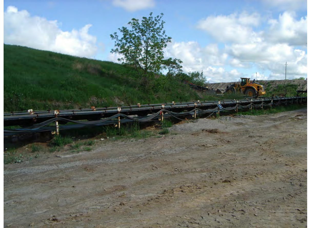
Photo 8: Second view of the conveyor. The berm is grassed and contains scattered trees and shrubs (mapped as Unit CUM1-1b on Figure 5. This portion of the berm and the yard in the foreground is within the proposed SPA extraction area. GEC 2022-05-28
